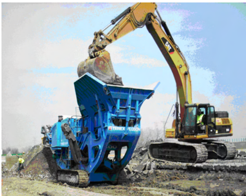
Concrete pavement being recycled on site with portable crushers for reuse in new pavement section on the South Tri-State (I-294)
