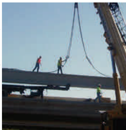
Concrete beams being installed at the U.S. Route 20 Bridge
