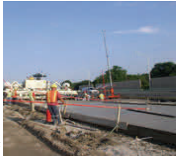
Crews smooth out newly poured concrete on the South Tri-State
