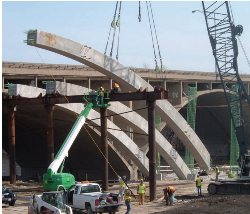
Concrete beams being installed for the new Fox River Valley Bridge.
