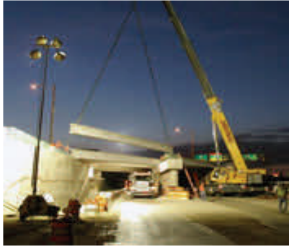
Bridge beams are erected during off-peak hours on the Central Tri-State Bridge over River Road
