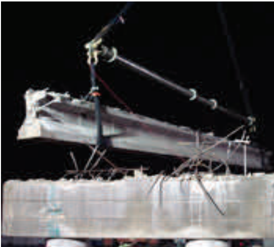
Removing concrete beams from the Kelley Road Bridge on the North Tri-State
